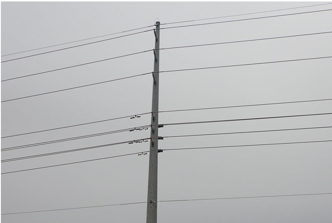
Closer detail of pole approximately 175' north of proposed structure
